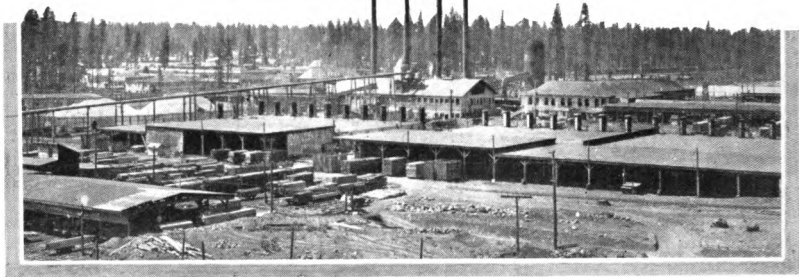
Power house, saw mill and kilns, store and administration building of the Red River Lumber Co., Westwood, Cal.
