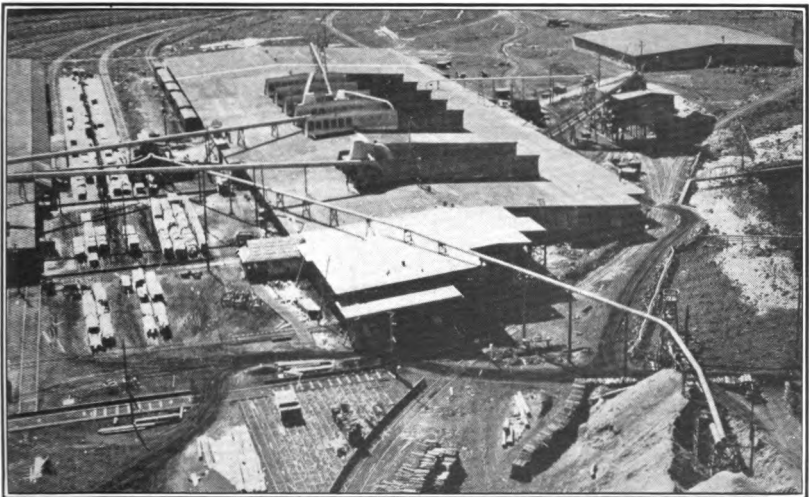
Blow-pipe system of the Red River Lumber Co., Westwood, Calif., extending from saw mill and box factory to saw dust pile.
